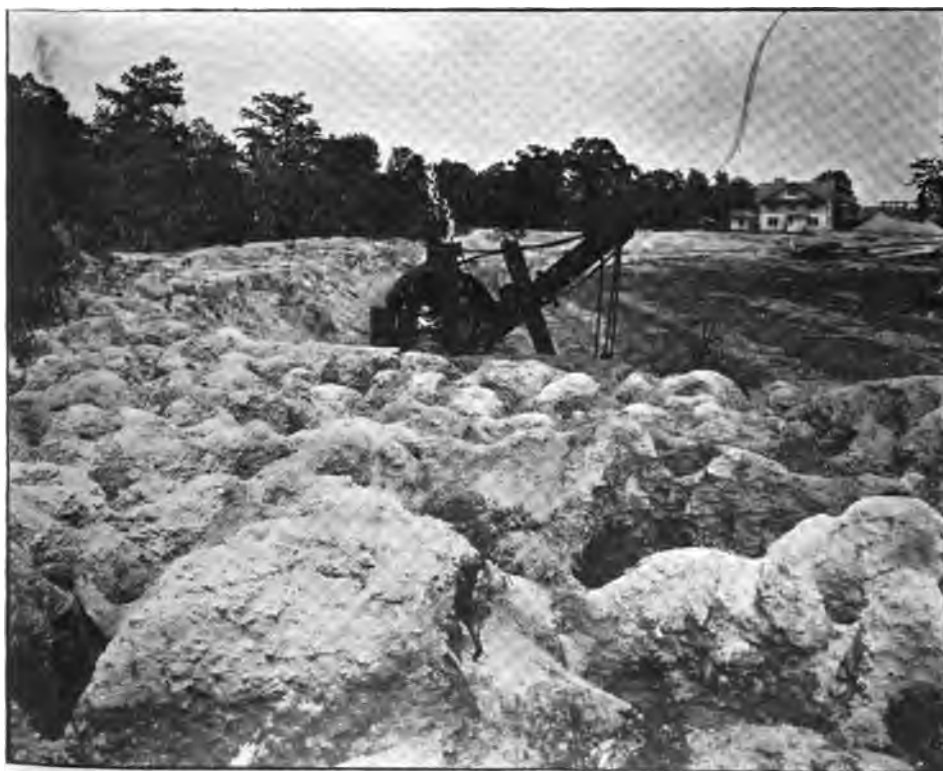
B. Fifty-ton steam shovel doing the work of fifty men.—Trent River Marl and Lime Company
